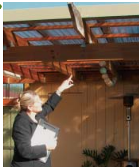
Cadet Building Surveyor Jeanette Gage inspects a new pergola. If you are building or replacing a roof on your home, verandah, patio or shed, please contact a qualified plumber to undertake the roofing.
